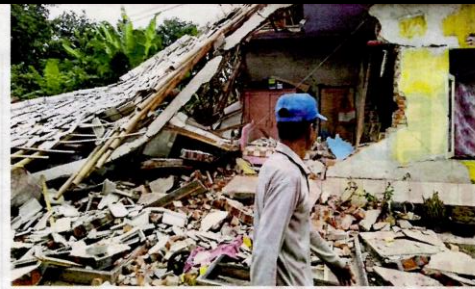
A man looking at damaged houses following an earthquake in Selong, Lombok, yesterday. AFP PIC
